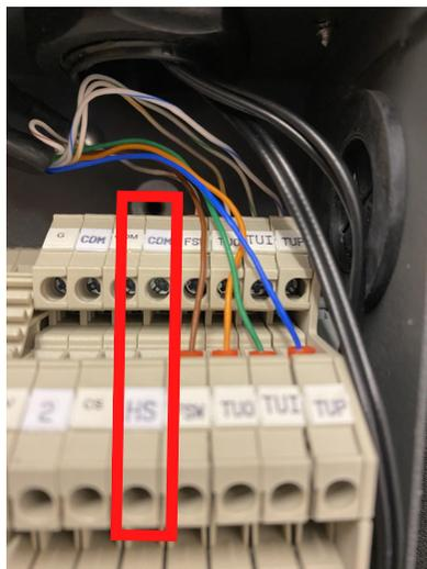
For external controls your call for heat should go into hs and com (neutral into com).
