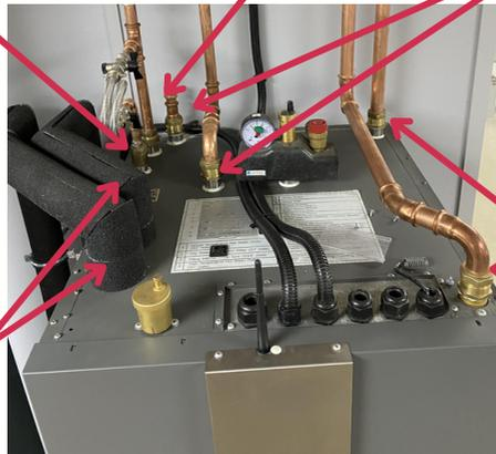
Two 1" male connections for heating/cooling side
