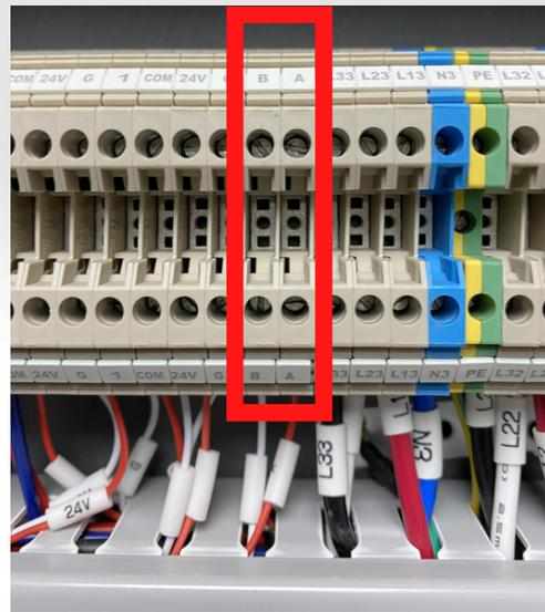
These are the connections for the supplied communication cables that go between the fan unit and indoor unit. please ensure they match on both units i.e FSW - white orange / orange, TUP - white green / green, TUI - white blue / blue, TUO - white brown / brown. The Grey communication cable is labelled A and B and should match on the indoor and outdoor unit.
