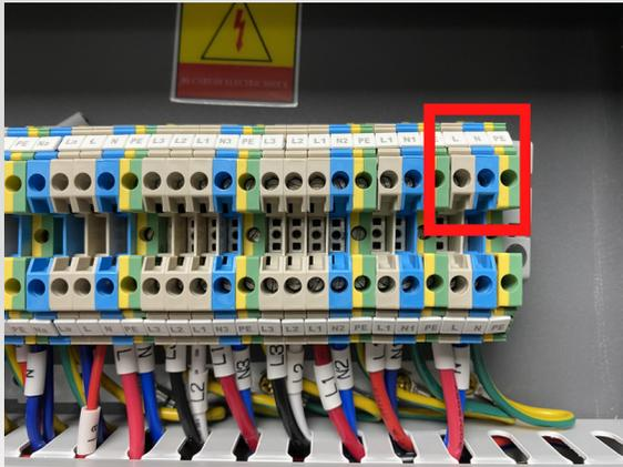
This is the connection for the power supply to the indoor unit. L / N / E
