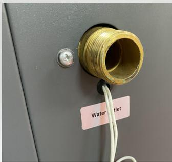
The outdoor unit has two 1" male connections, the top connection is the flow to mono unit and bottom is return
