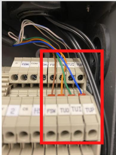
These are the connections for the premade cable that goes between the heat pump and indoor unit
