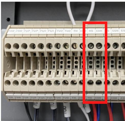
For external controls your call for heat should go into "hs" and "com" The neutral wire from your heating controls should be connected into com.
