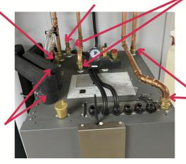
Two 1" male connections middle and high temp hot outlet
