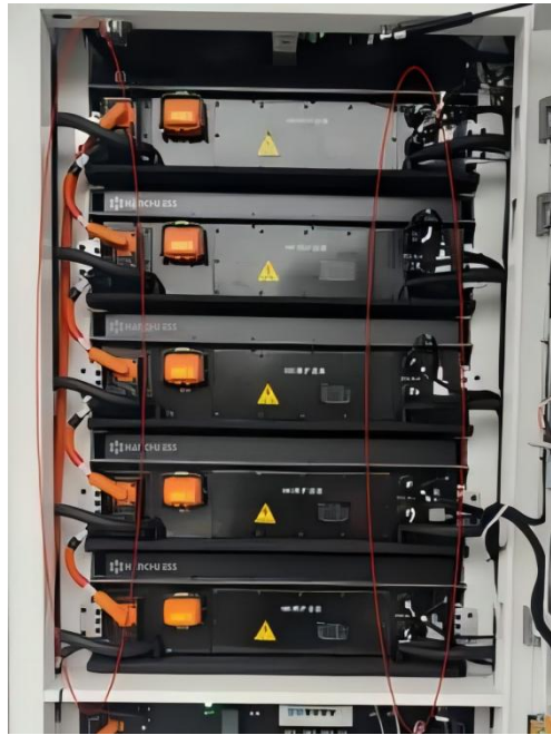
Figure 8-6 Cooling Pipe&amp;Valve Position
